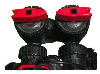
When the red handles are pointed at each other you have successfully bypassed the unit. The water is no longer being treated.
